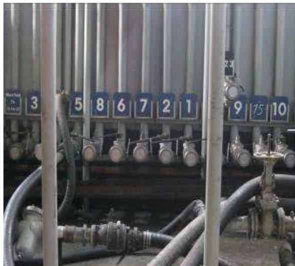
**Figura 46: Despacho a Camión Cisterna de Productos a Granel**
